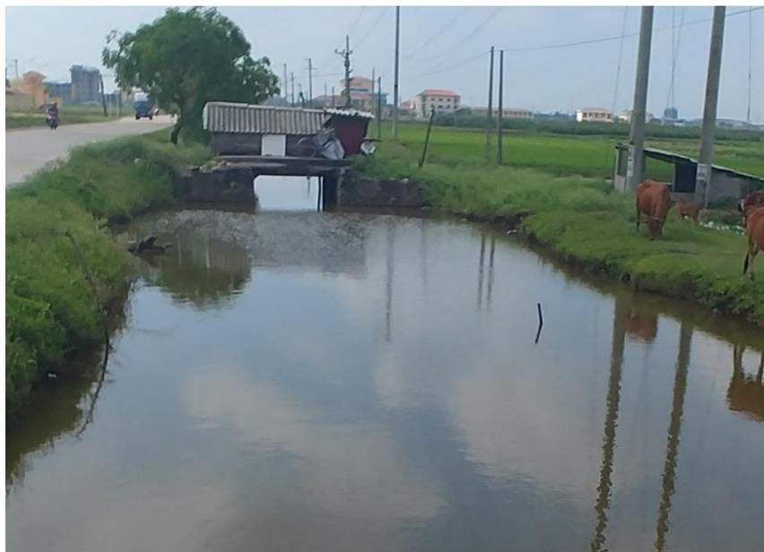
**Figure 14** Section flow reduced by a self-made bridge
